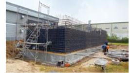
Construction of a fire extinguishing tank for the sprinkler system
