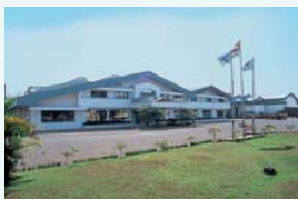
PT. LINTEC INDONESIA
