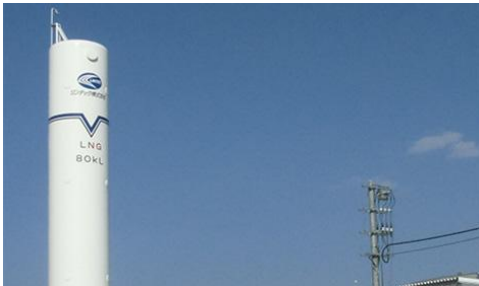
Satellite facility at Komatsushima Plant
