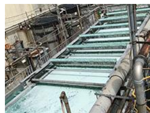
Effluent processing equipment at the Kumagaya Plant
