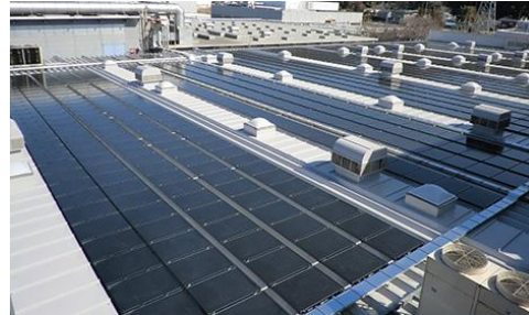
Solar panels at the Agatsuma Plant (about 5,000m 2 )
