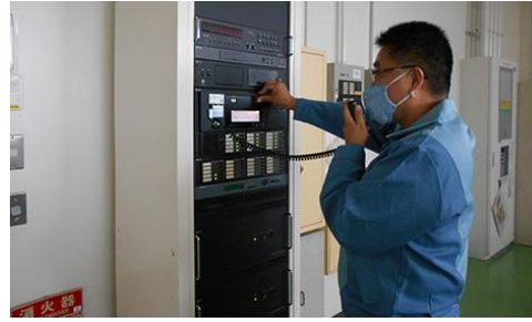
Exercise for emergency broadcast procedures in the event of power outage (Chiba Plant, March 2021)
