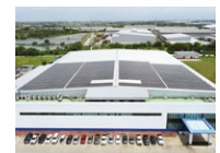
Panel fotovoltaik dipasang
