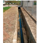
Completely cleaned gutters
