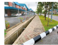
Zebra pattern we repainted
