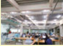
LED lighting after replacement
