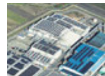
Solar panels at the Doi Plant (about 10,000 m 2 )
