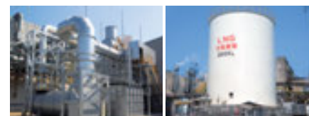
Measures to reduce environmental impact Left: Waste heat boiler at the Doi Plant Right: LNG satellite facility at the Mishima plant
