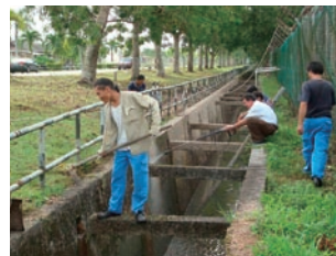
Cleaning a waterway near the plant
