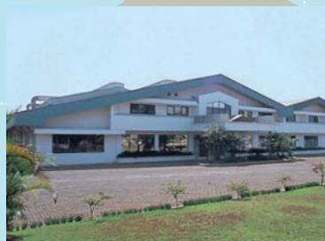
PT. LINTEC INDONESIA
