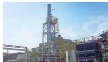
Gas engine cogeneration system introduced at the Kumagaya Plant
