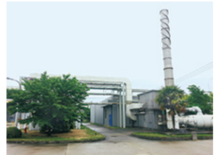
External appearance of a plant with enhanced environmental protection
