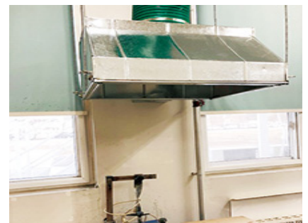
Installed exhaust pipe
