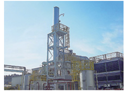
Gas engine cogeneration system introduced at the Kumagaya Plant
