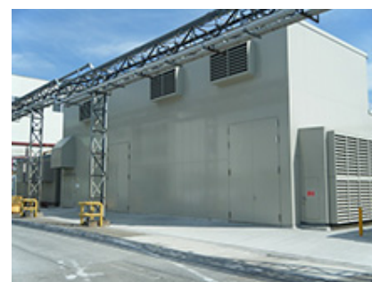
Non-utility generation facility at Kumagaya Plant
