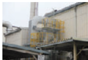
An economizer installed at an incinerator boiler (Tatsuno Plant)
