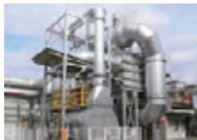
Waste-heat boiler installed in the Shingu Plant
