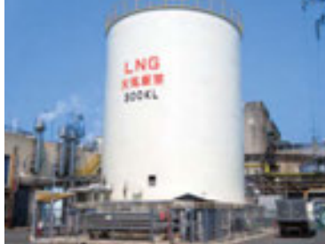
LNG satellite facility at the Mishima Plant
