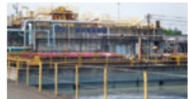
Effluent treatment facility at the Kumagaya Plant
