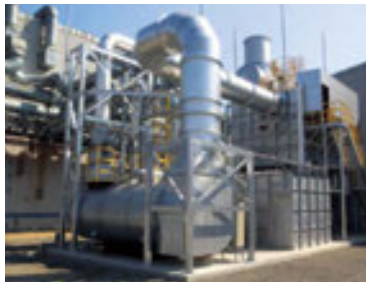
Waste heat boiler at the Doi Plant
