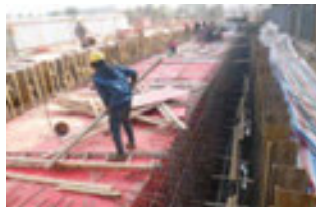
Construction of an emergency wastewater tank for preventing discharge
